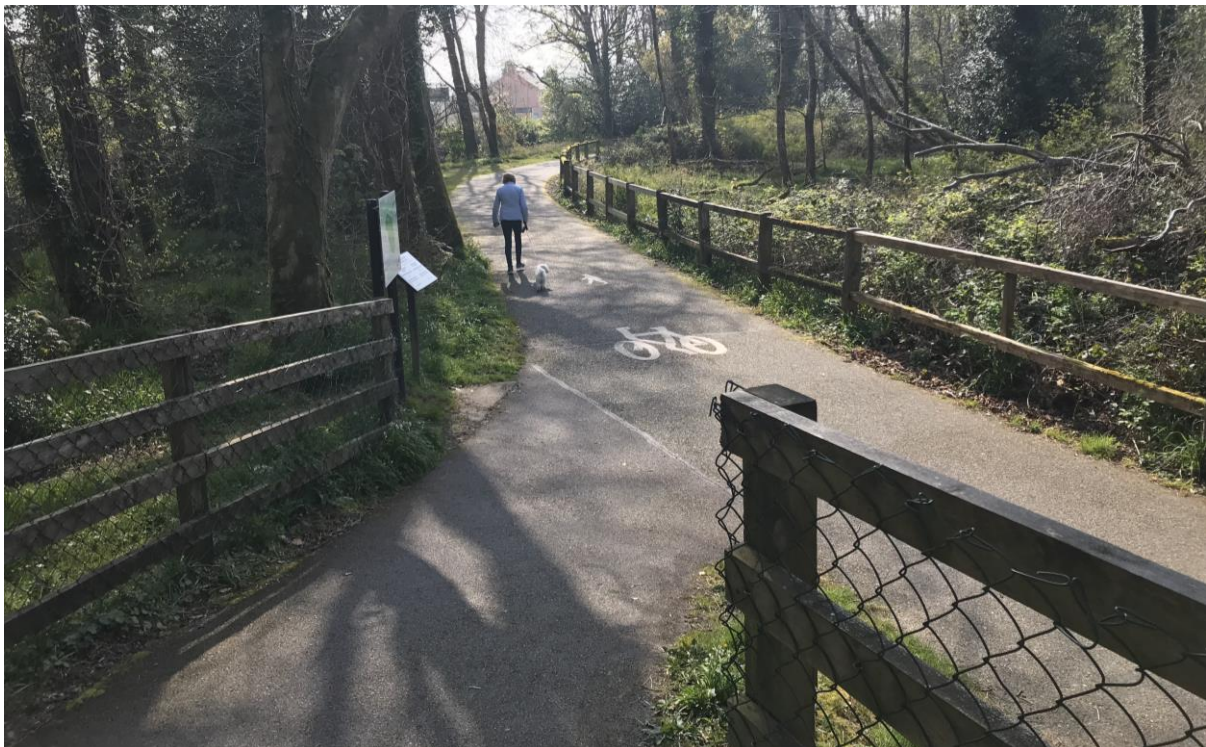
Figure 17.1 Existing Off road shared facility in Killarney National Park opposite site entrance
